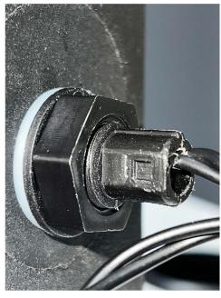
**Step 2** On the back side of the tank there will be a bung needing a plug. Using one of the supplied plugs, apply the supplied thread sealer and tighten until snug.
